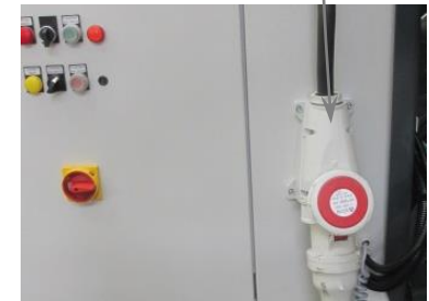
ep+: Socket for external power supply
