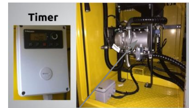
HEATING SYSTEM FOR LUBE OIL TANK
